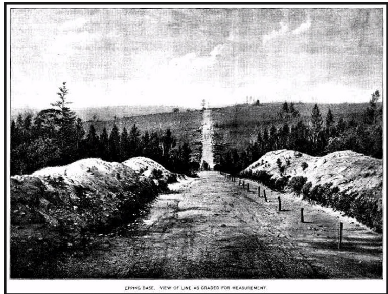
Epping Baseline Construction - In order to map the Atlantic seaboard for navigation and national defense in the early 1800's using a chain of triangles, six baselines were constructed from Maine to Louisiana, measured and built with extreme accuracy. In 1857, local farmers and lumbermen were hired to grade a 12-foot-wide path along the 6th and final baseline, located in Downeast Maine. Photo source: geocaching.com.
